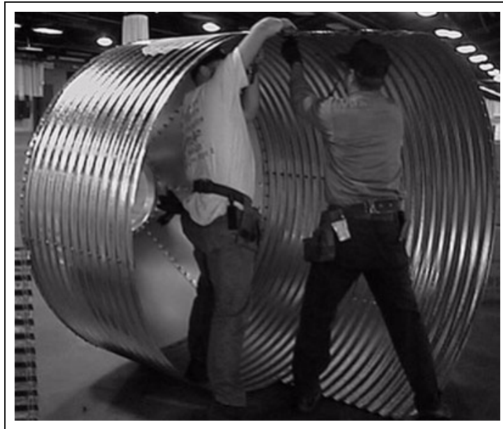
Figure 6F Sidewall Assembly
